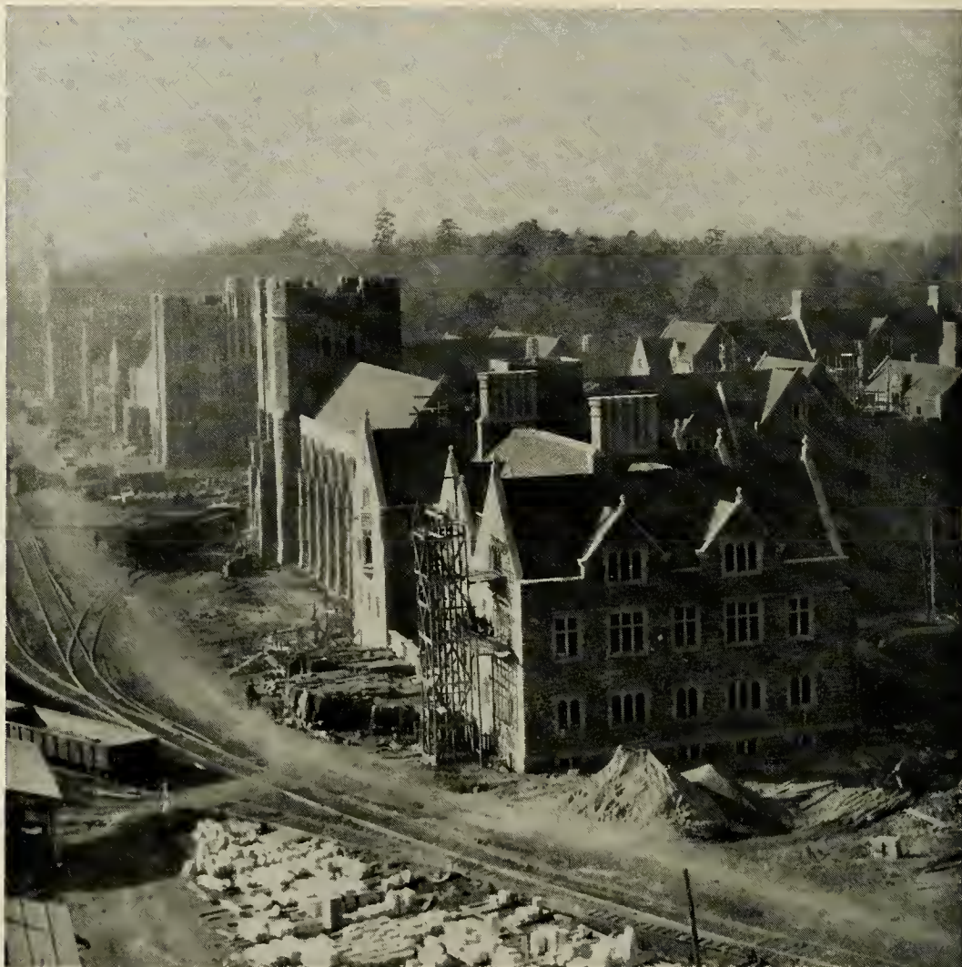
Duke had its own railroad during construction of the University's West Campus, when temporary railroad tracks ran the length of the main campus for trains that hauled stone and other building materials.
